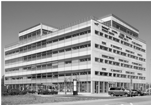
Figure 4.X South and East façades of Kaggen in Malmö (photo: Rafael Palomo).
